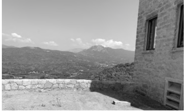
Picture before : metric survey
