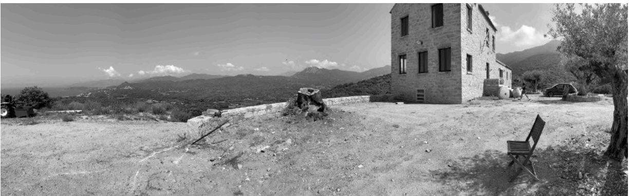
Picture before : metric survey
