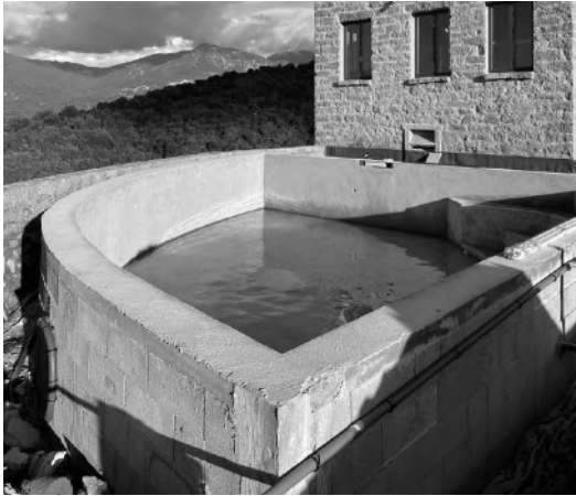
Pictures of the construction
